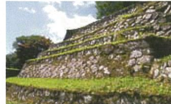
1 The ruins of Iwamura Castle The stone walls extend about 1.7km. About 40,000 stones are piled up. You can see three ways of piling up stones.
