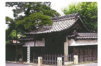
2 The ruins of Oi-juku Honjin Although most of the building was burned in the fire, the gate and pine trees which survived the fire recalls of the prosperity of Oi-juku.
